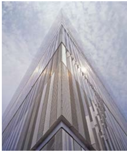
Grids made of triangular stainless-steel rods lend structure to the panels on the base of 7 World Trade Center. Like the entire building envelope, this facade also consists of two layers.
